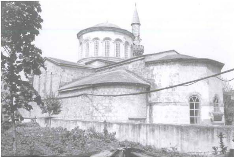
5 St Eugenios from the south-east. The string moulding around the main apse copies that at Hagia Sophia. The original porch by the south transept was removed, probably when the church was converted into a mosque
